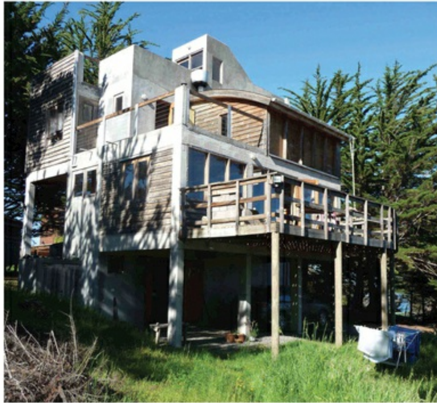
FIGURE 3.2.B The Keller Home in Pichilemu, Chile
