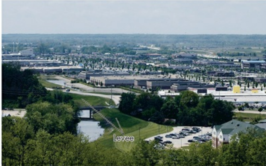
FIGURE 6.22 Development Increases on St. Louis Area Floodplains
