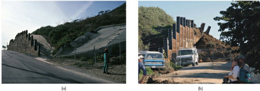
FIGURE 7.33 Retaining Wall Built Following the 1995 Landslide
