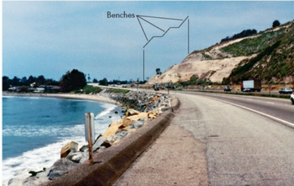
FIGURE 7.26 Benches on a Highway Roadcut
