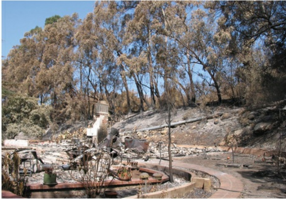
FIGURE 13.6A Home Lost during the Santa Barbara Jesusita Fire of 2009 The fire raced up Rattlesnake Canyon, claiming more than 10 homes. This home had large eucalyptus trees just upslope that burned extremely hot and most likely contributed to the loss of the home. (Edward A. Keller)
