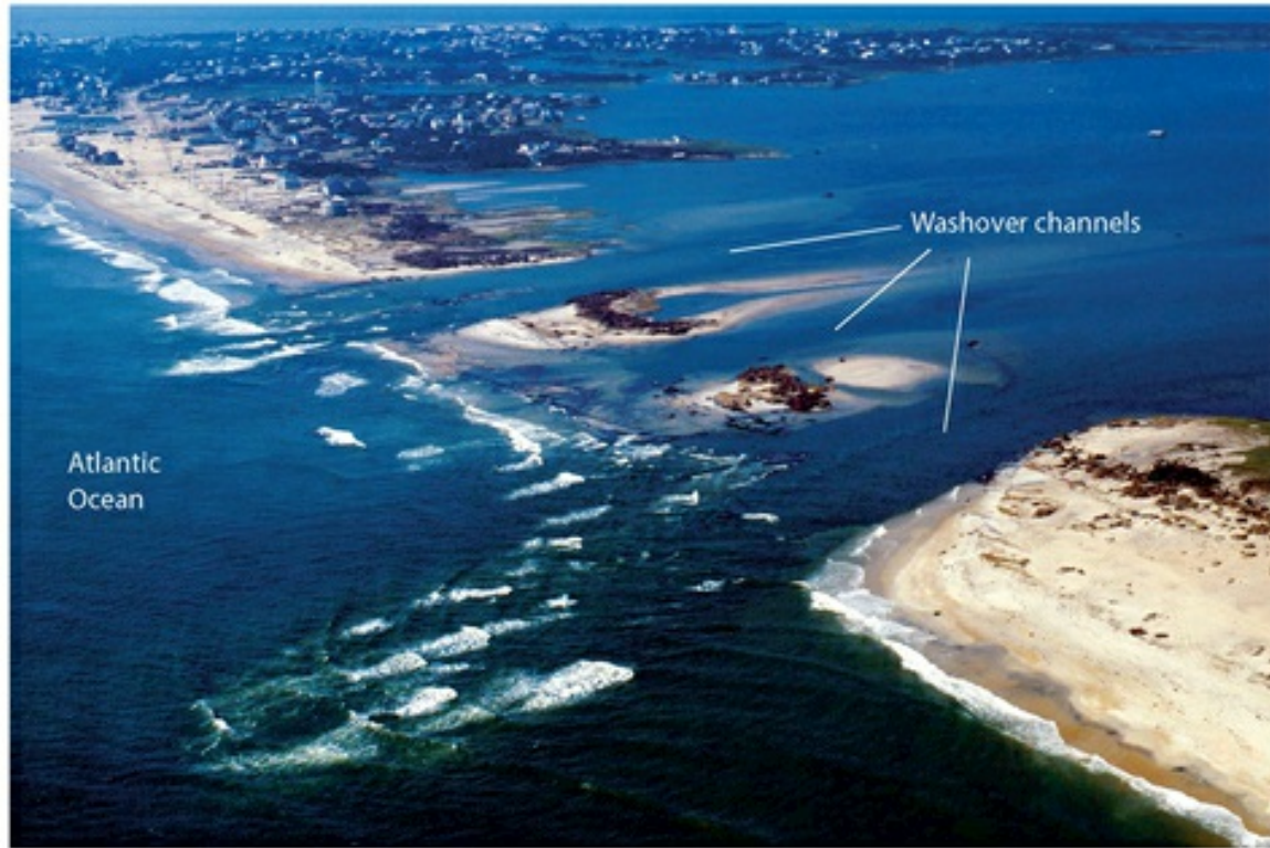
FIGURE 10.21 Hatteras Island Breached by Hurricane Isabel Storm Surge Three channels, totaling 500 m (~550 yd.) in width, were cut through Hatteras Island, North Carolina, by Category 2 Hurricane Isabel in September 2003. The breach, located close to where the eyewall crossed the island, is just west of Cape Hatteras. These washover channels were created by a 2.3 m (~7.6 ft.) storm surge in the right forward quadrant of the storm. (USGS)
