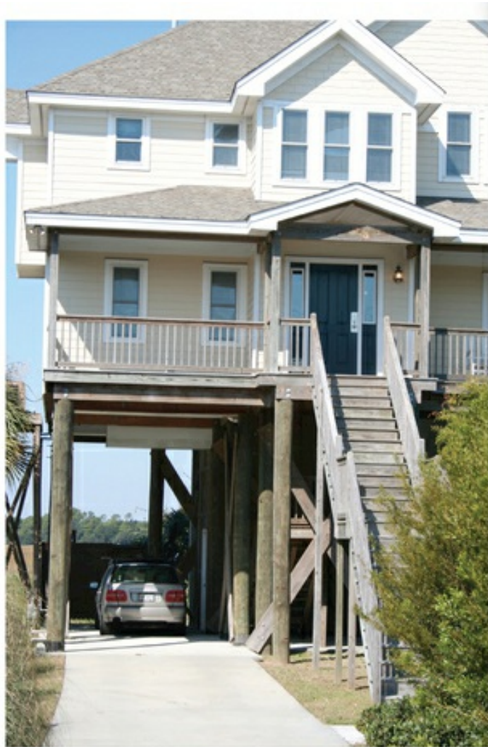
FIGURE 11.34 New Home Construction on Folly Island
