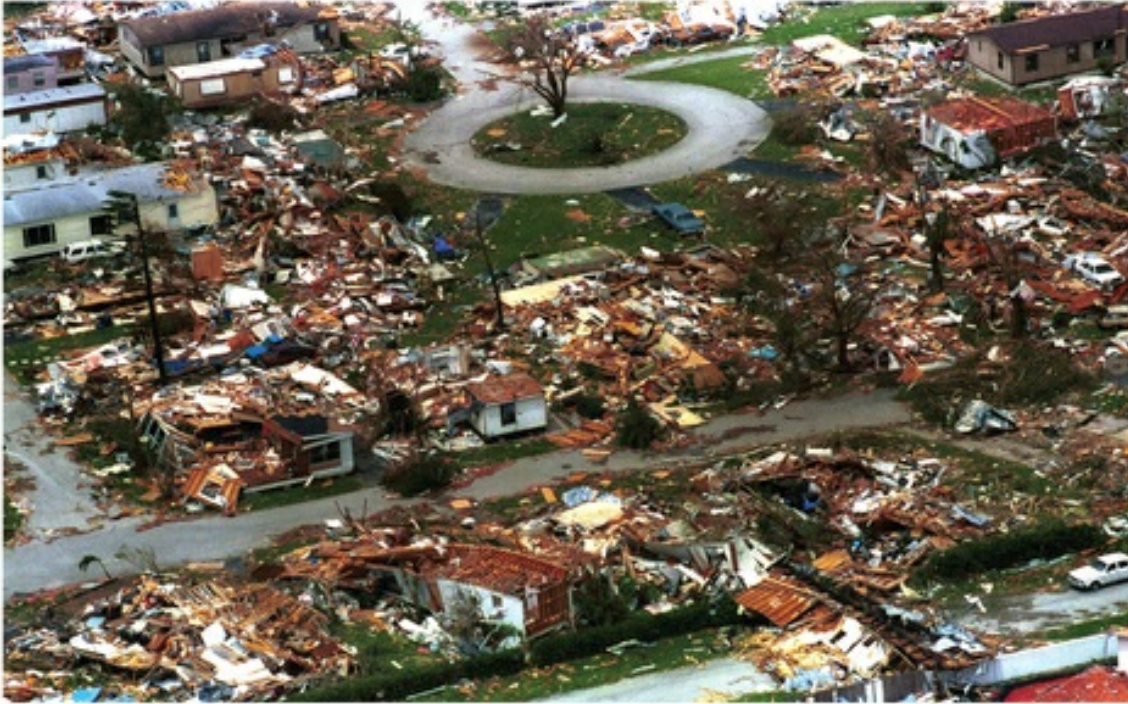
FIGURE 10.22 Aerial View of Hurricane Wind Damage
