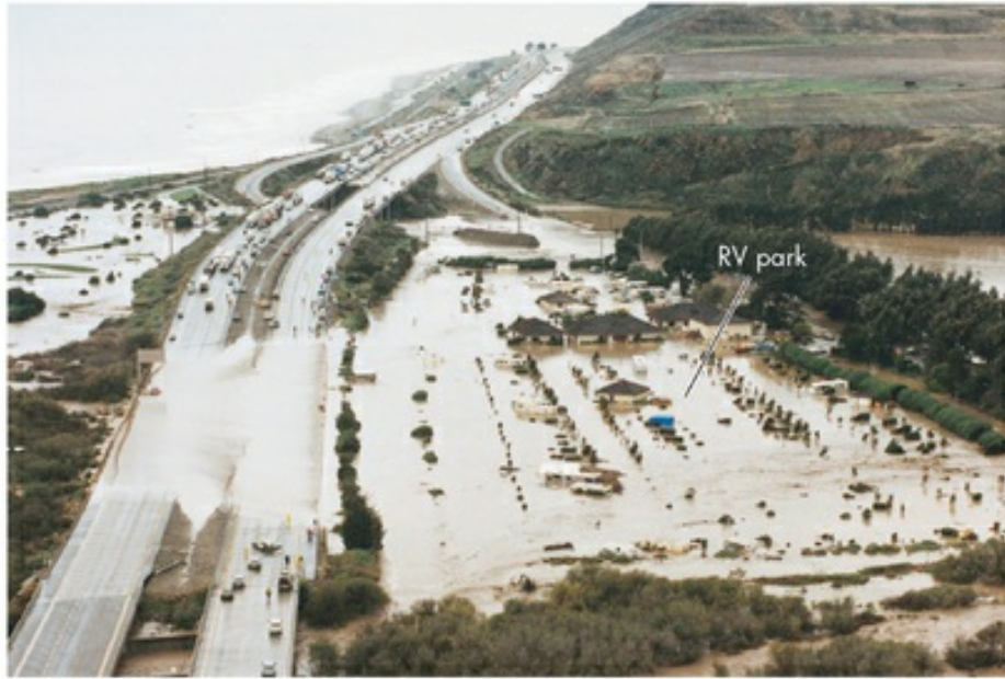
FIGURE 6.23 Flooding of California's Ventura Beach RV Resort in February 1992 The RV park was built directly across a historically active distributary channel of the Ventura River Delta. The recurrence interval of this flood is approximately 22 years. A similar flood occurred again in 1995. On the left, U.S. 101, the Pacific Coast Highway, is completely closed by the flood event. (AP Photo/Mark J. Terrell)
