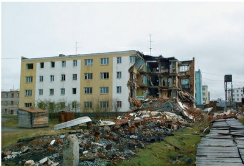
FIGURE 8.24 Melting Permafrost Destroys Building
