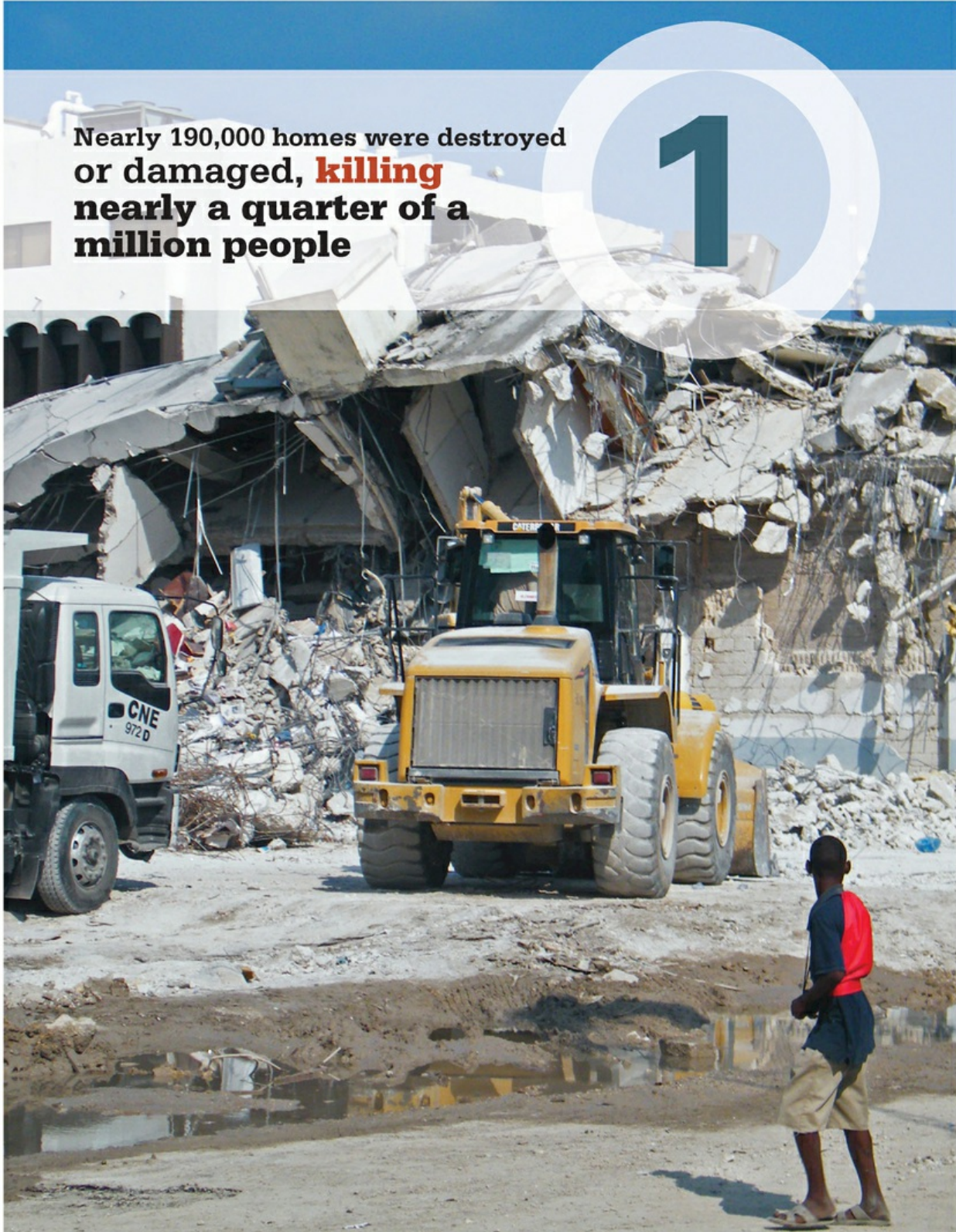
Collapsed buildings in Port-au-Prince, capital of Haiti, resulting from the January 12, 2010, earthquake that killed more than 200,000 people. The extensive damage and loss of life were in part a result of the high population density in the capital and poorly constructed buildings unable to withstand the earthquake shaking. (Tommy E Trenchard/Alamy)
