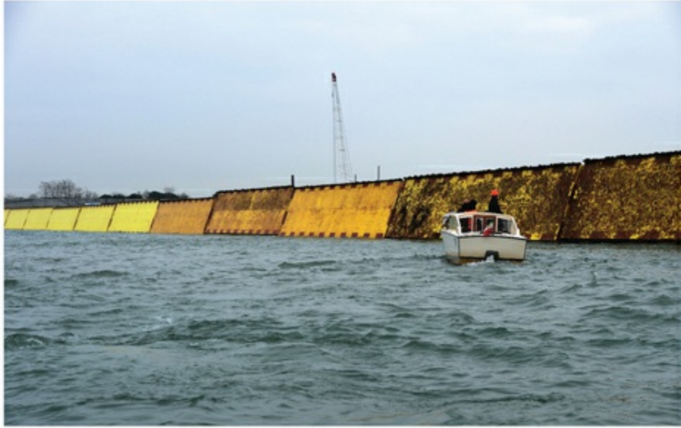
FIGURE 8.35 Flood Control Structures During Construction (©Getty Images/VINCENZO PINTO/Staff)
