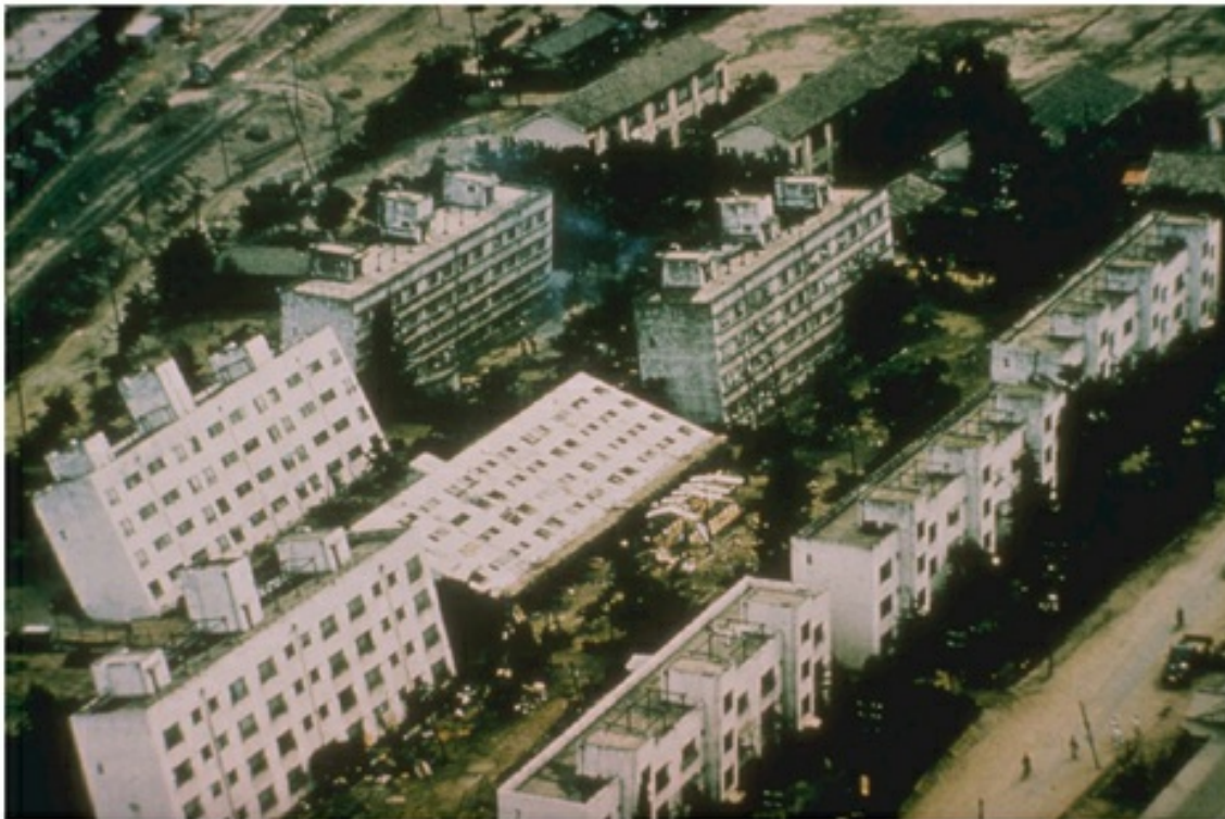
FIGURE 3.28 Building Collapse from Liquefaction
