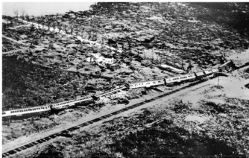
FIGURE 10.23 Hurricane Blows Train off Tracks in Florida Keys
