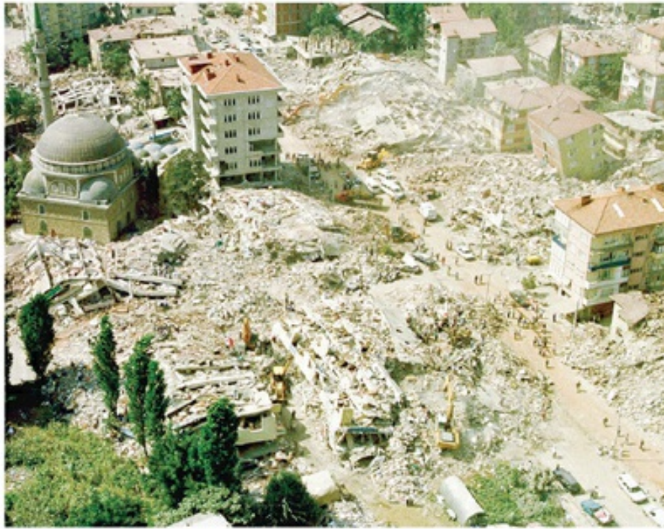
FIGURE 3.36 Collapse of Buildings in Turkey Damage to the town of Golcuk in western Turkey from the M 7.6 Izmit earthquake in August 1999. The very old mosque on the left remains standing, whereas many modern buildings collapsed. (AP Photo/Enric Mariti)
