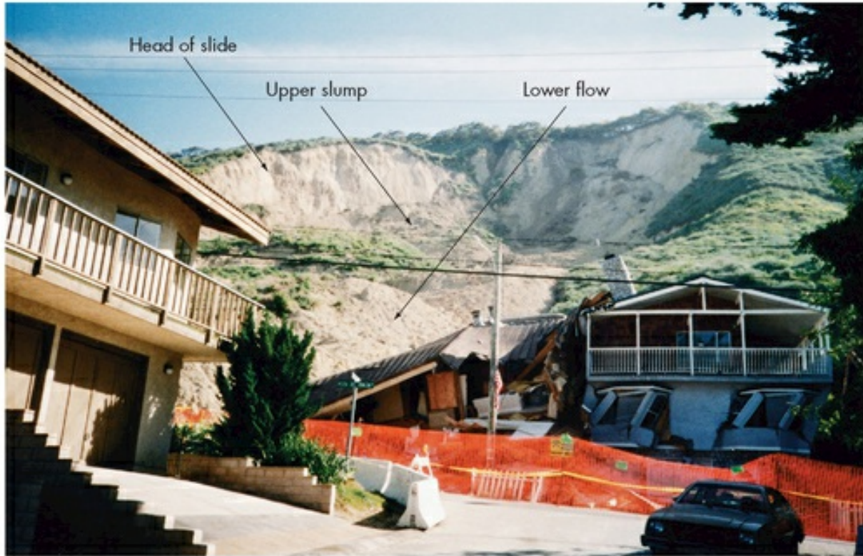
FIGURE 7.6 Houses Buried by Complex Landslide
