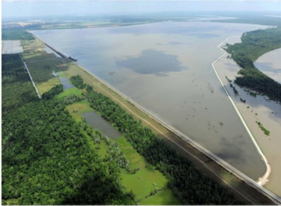
FIGURE 6.37 Mississippi River Levee
