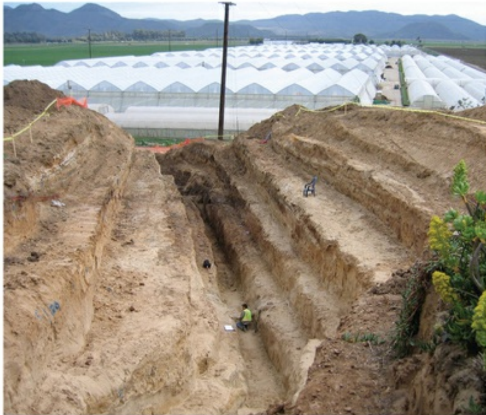
FIGURE 3.6 Paleoseismic Trench Photograph of a paleoseismic trench excavated across folded sediments above a blind fault in Southern California. (Duane E. DeVecchio)
