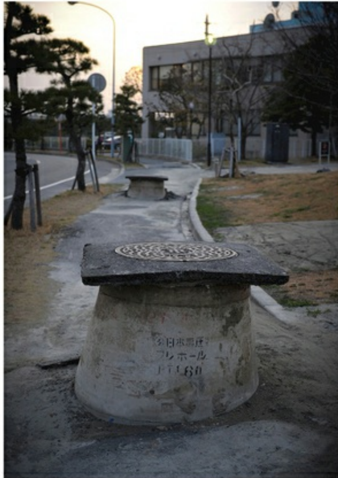
FIGURE 3.41 Damage Due to Liquefaction Manholes to underground sewer system forced through overlying sidewalks due to ground surface subsidence (lowering) caused by liquefaction. (Koki Nagahama/Getty Images)
