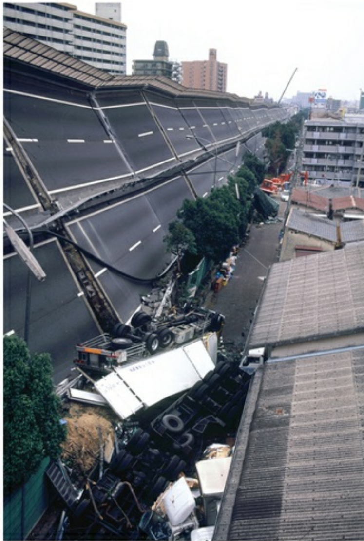
FIGURE 3.38 Damage from 1995 Kobe Earthquake
