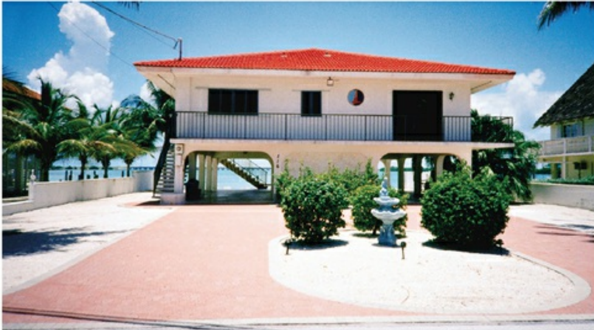
FIGURE 10.27 Hurricane-Resistant House Home in the Florida Keys that has been constructed with strong blocks and space below the living area to allow a hurricane storm surge to pass through the building. (Edward A. Keller)
