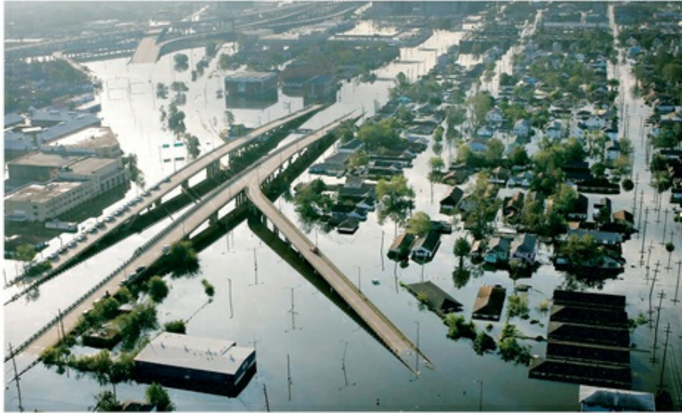
FIGURE 10.14 New Orleans Inundated after Flood Protection System Fails
