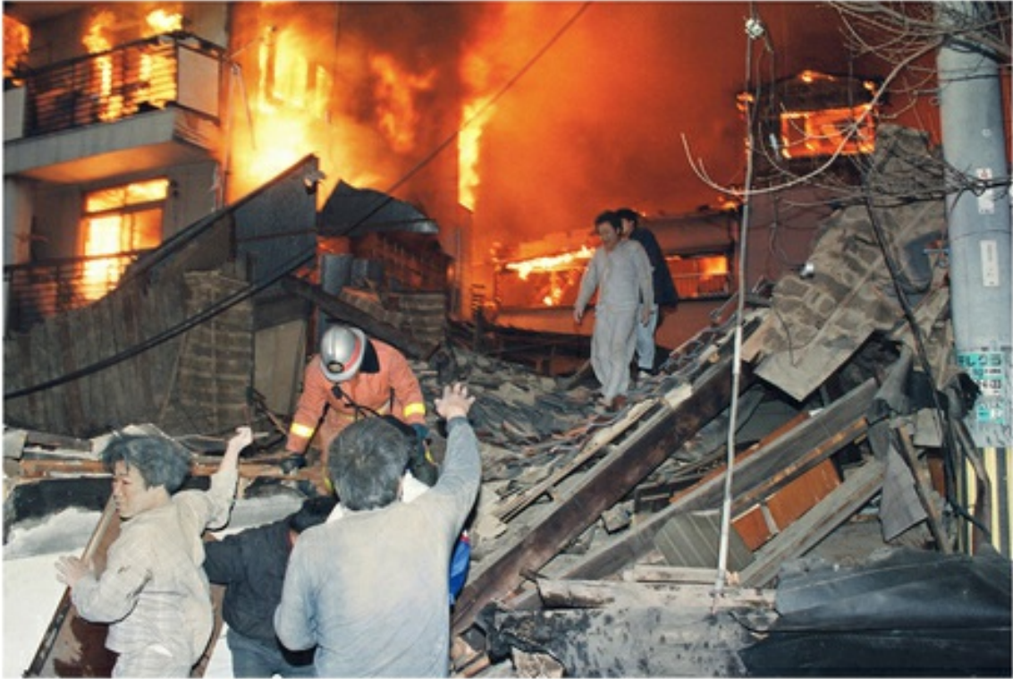
FIGURE 3.30 Earthquake and Fire Fires associated with the 1995 M 6.9 Kobe, Japan, earthquake caused extensive damage to the city. (©Getty Images/The Asahi Shimbun/Contributor)
