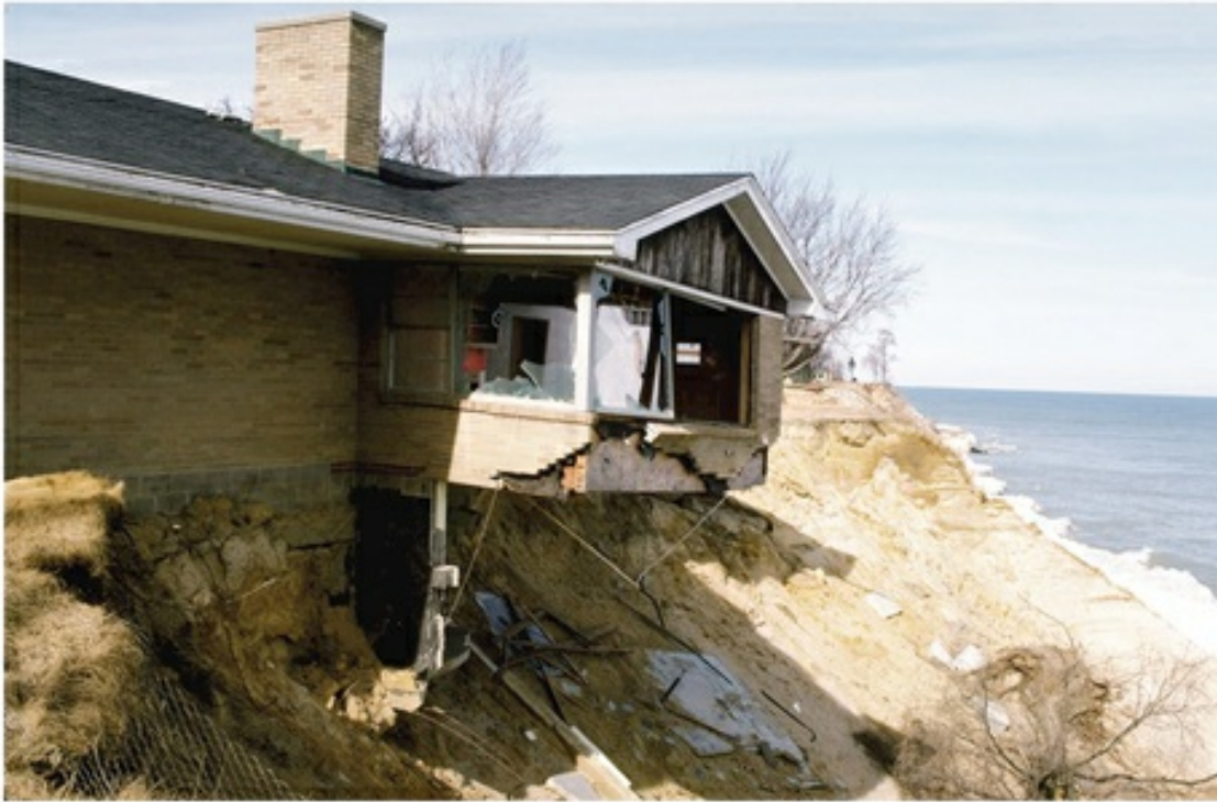
FIGURE 11.21 Lakes Have Coastal Erosion Problems Coastal erosion along the shoreline of Lake Michigan has destroyed this home. (Steve Leonard)
