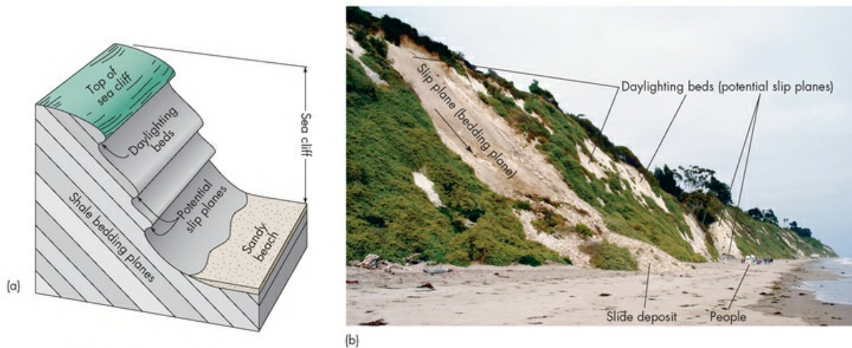
FIGURE 7.7 Daylighting Beds (a) Bedding planes that intersect the surface of the land on a slope are said to "daylight." Such beds are potential slip planes. (b) This slide occurred in late 2003. Failure was along a daylighting bedding plane. Slide deposits cover part of the beach. (Edward A. Keller)
