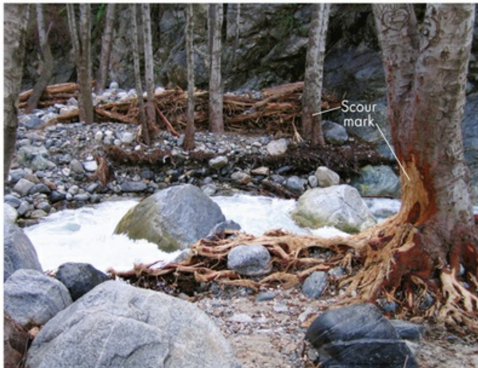
FIGURE 6.48 Scour Marks Indicate Flood Height
